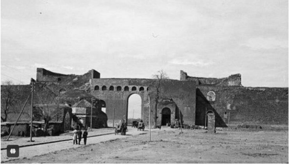
Figure 2. Diyarbakır Walls (Old Urfa Gate) (Antoloji Diyarbakır, 2024).
